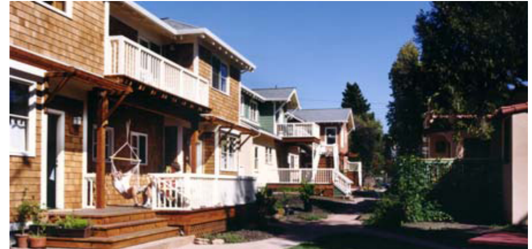
Berkeley Cohousing used a 15% fly ash concrete mixture as their foundation for all of their housing units, as well as their common house
