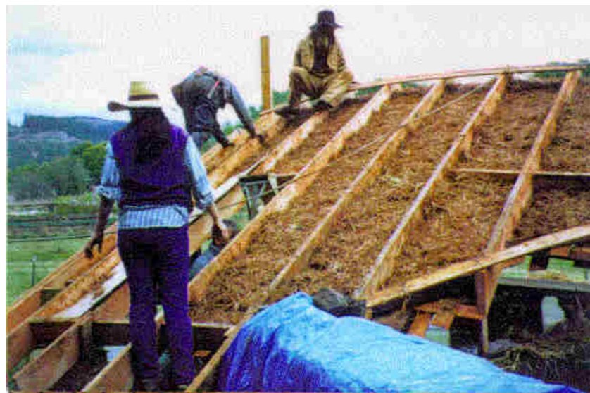
Straw/Clay Composite with Wood Structure
