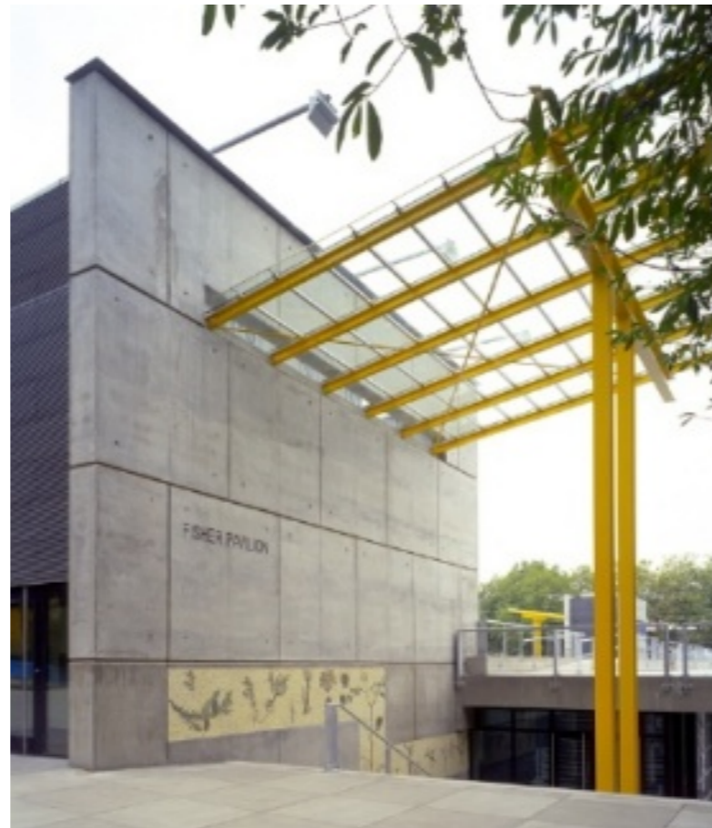
Fly Ash Concrete
