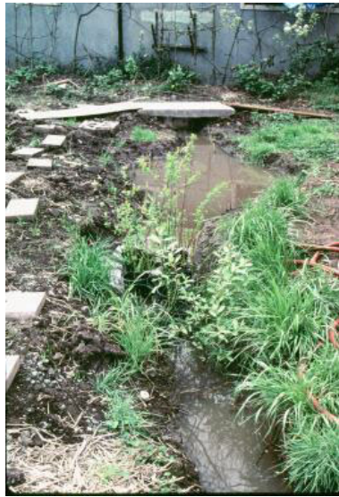
Rainwater catchment swale that meanders through site
